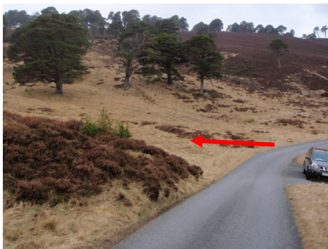
Fig. 2 : Start of new access (north)
